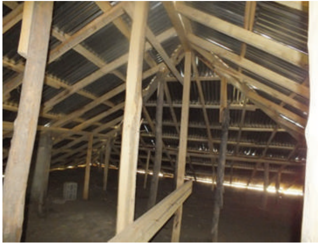
Fig. 13-25. Wooden roof implementation.
