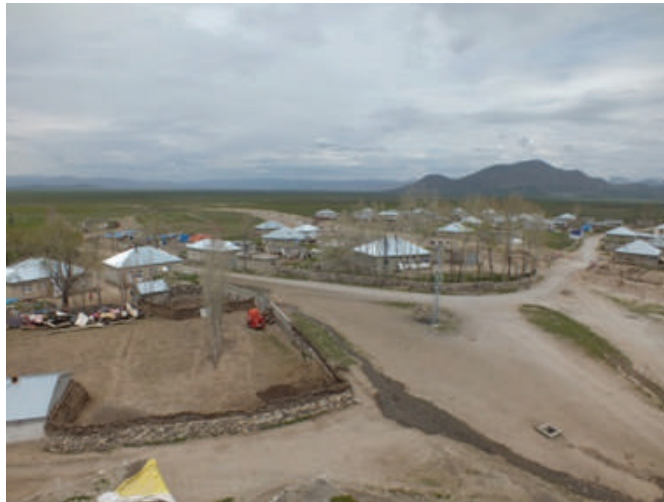
Fig. 13-21. Structures in the residential area.
