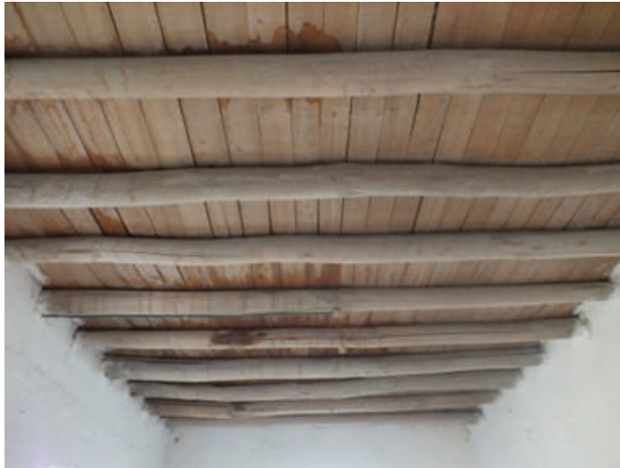
Fig. 13-24. Top flooring implementation.
