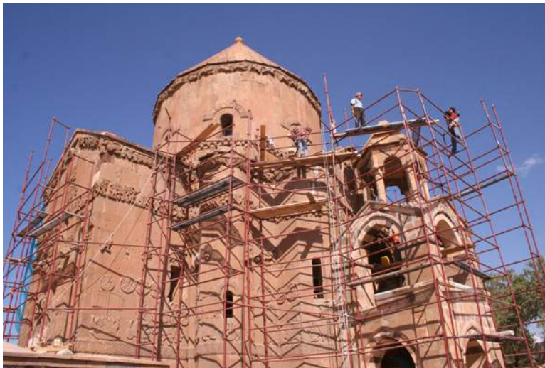
Fig. 3-9. Scaffolding, photographed by Uğur Kartav
