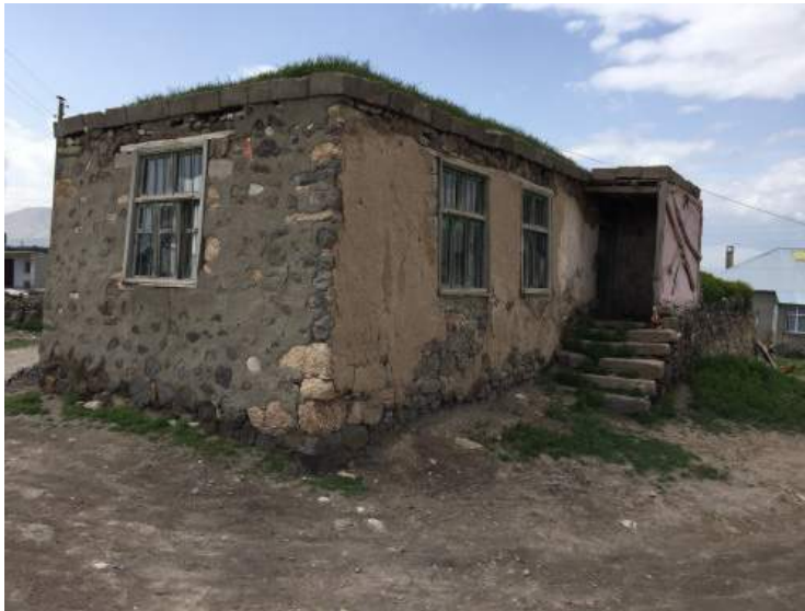
Fig. 13-22. Structures in the residential area.
