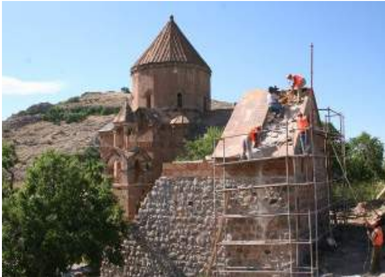
Fig. 3-4. A scene of restoration process.
