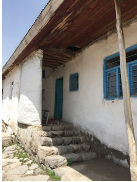
Fig. 13-27. Entrance area of a dwelling.
