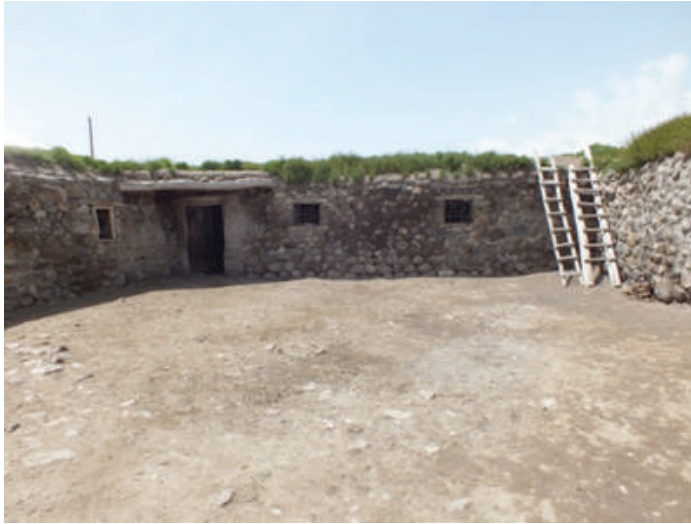
Fig. 13-18. The courtyard surrounded by the units.
