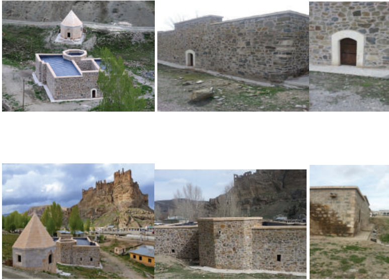
Fig. 6-6. Views of Evliya Bey Madrasa after renovation, photos by Architect Hakan İrven
