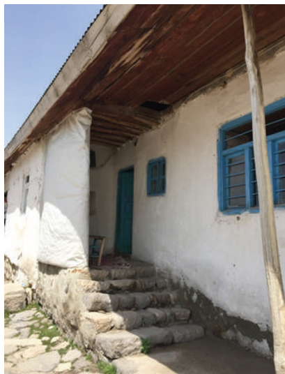
Fig. 13-20. Entrance area of a dwelling.
