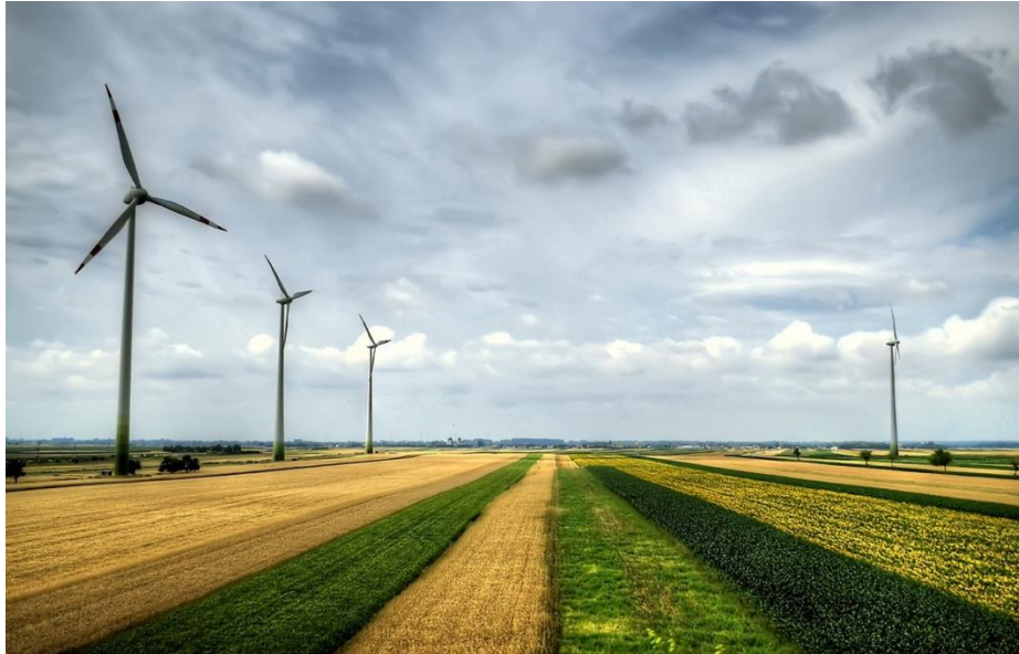
Figure 5: Sample of Wind farm [22]
