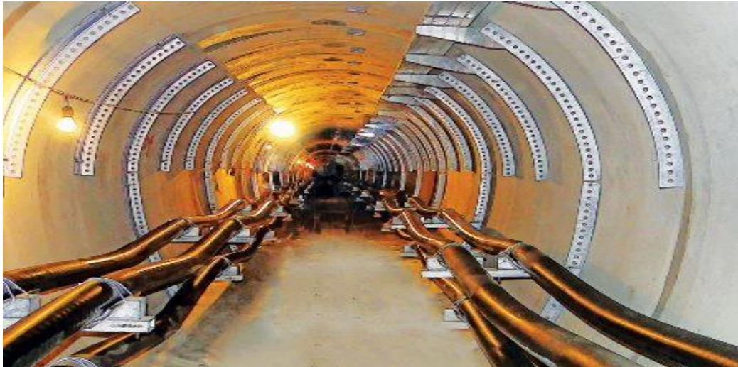
Figure 3: Underground Transmission lines [23]
