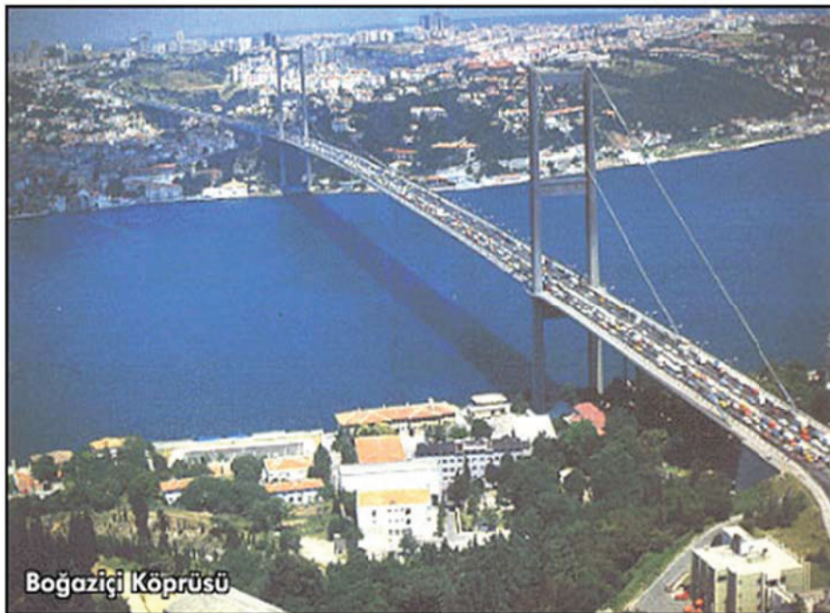
Figure 2 : A general view of Istanbul Bogazici Bridge
