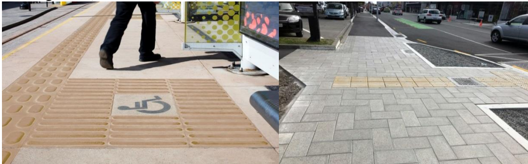
Rehber yol yüzeyi, Buff; Directional tactile indicators (Ann-Marie Head) (Waka Kotahi NZ Transport Agency, 2023)
