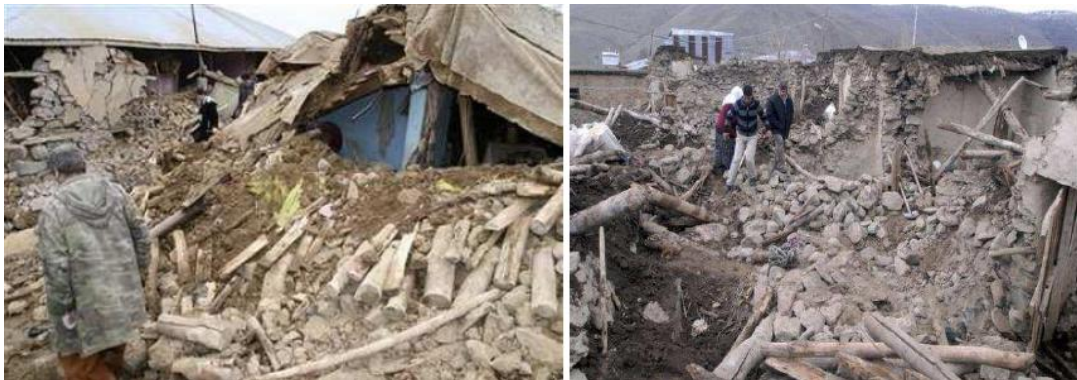
Figure 11. Destroyed adobe buildings in Elazığ earthquake [27]
