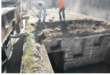
Figure 14. Took down roof
