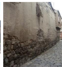
Figure 10. The moisture problems
