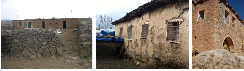
Figure 12. Type of window use in architecture of the rural region, Diyarbakır, 2012, photographed by author
