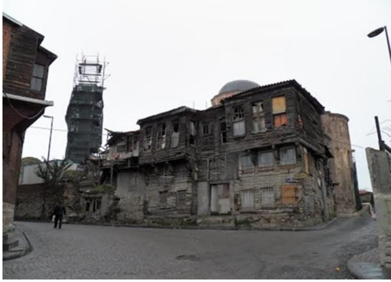
Figure 10. Decay in Zeyrek [8]
