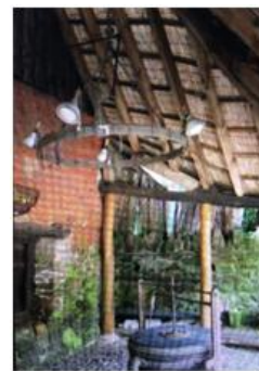
Figure 17. View of a reed roof structure [22]
