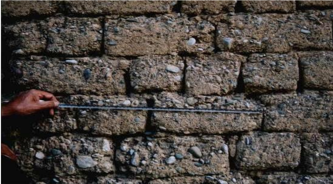
Figure 8. A view of a wall made of adobe material which consists of big aggregate [22]
