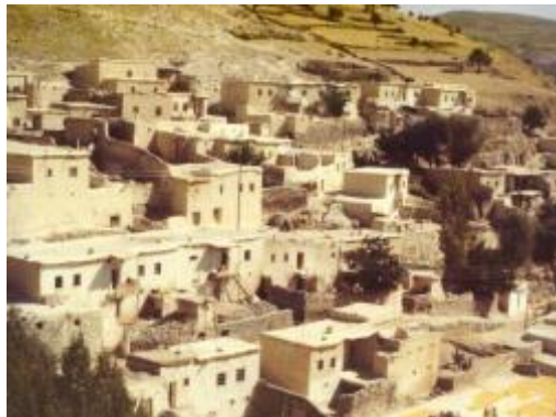
Figure 3. Building settlement constructed from adobe material, Akçadağ [7]
