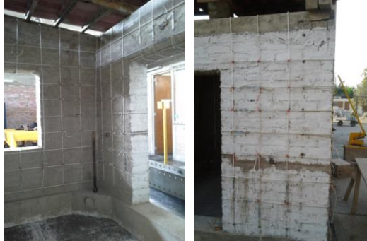
Figure 4. Nylon rope mesh provided to reinforce a full-scale adobe housing model to be tested on the shaking table. The nylon rope used had a nominal diameter of \frac{1}{4} ". The vertical ropes were placed through the bottom mortar layer and around the wooden crown beam. The horizontal ropes were spaced every two adobe masonry courses. Thinner nylon cross-ties (red ropes on the photos) were placed to join the mesh on both faces of the walls.
