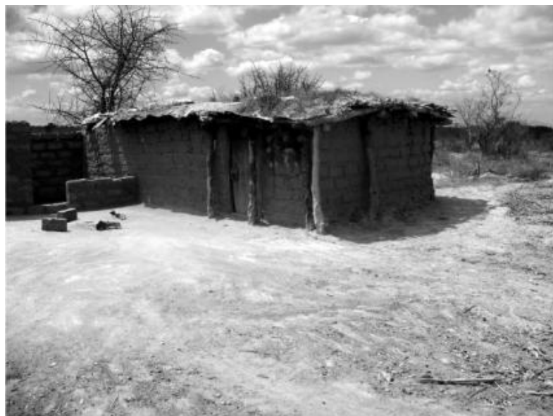
Figure 9. Plants growing up in an adobe house causes biological decays. Adobe constructed building in Dodoma, Tanzania [23]
