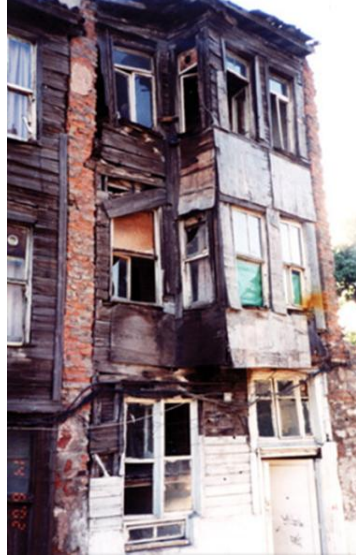
Figure 11. A ruined house in Zeyrek [8]
