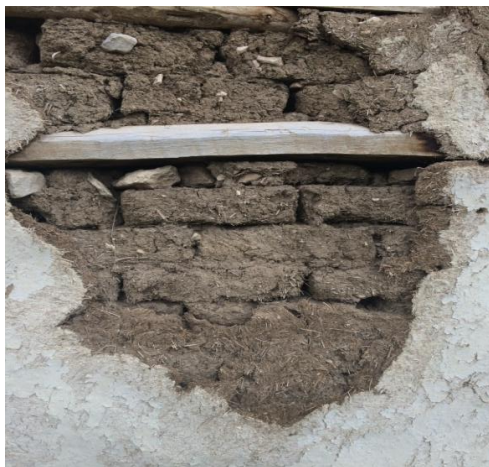
Figure 7. Since a periodical maintenance on the building was not done, the plaster and the paint of the building felt down
