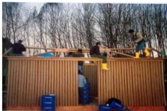
Figure 4. Rescuers Working to Prepare the Floor and Seats of Temporary Paper Homes in Turkey [9]
