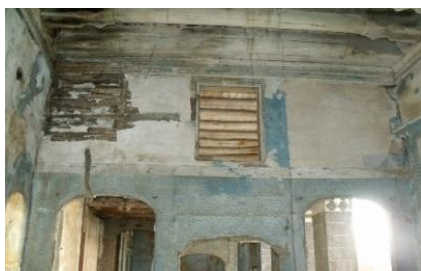
Figure 8. Some wood-adobe deterioration
