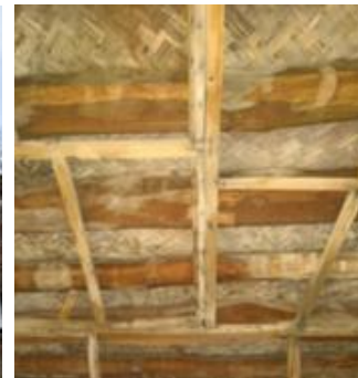
Figure 15. Structure and coating
