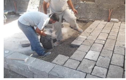
Figure 16. Paving with basalt stone
