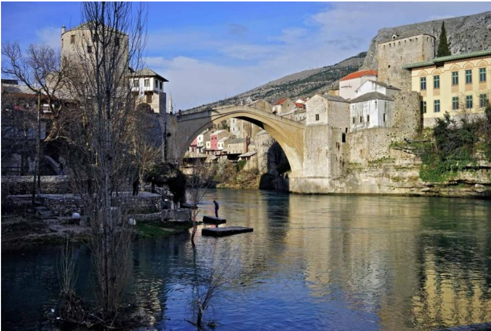
Figure 10. Bosnia, Mostar Bridge in 2004, photograph:Giles Clarke/Getty Reportage [19]
