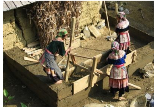
(b) An example of an adobe building in which mud is poured into a mold in Vietnam [9]
