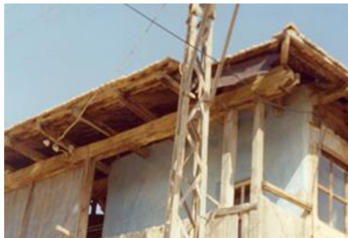
Figure 16. View of bearing rafters in a roof covering made using traditional techniques
