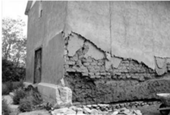
Figure 10. Damage in a structure with cement-based plaster [17]
