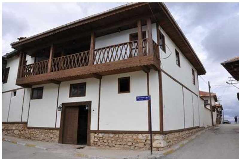
Figure 7. An adobe house with a rock foundation on Engin Sokak in the Kaş District of Yalvaç, Isparta [15]
