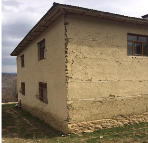
Figure 5. Decays caused by rain on the sides of the building with and without the effect of the wind
