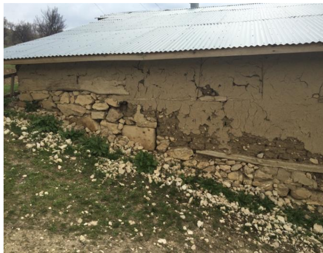
Figure 6. Decays caused by rain at the most outer plaster of the adobe building. The decays does not look aesthetic
