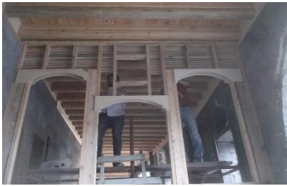
Figure 17. Adobe filled wood wall
