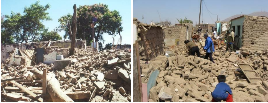
Figure 1. Total destruction of adobe houses caused by earthquakes in El Salvador (2001, photo by Dominic Dowling, left) and Pisco, Peru (2007, right)
