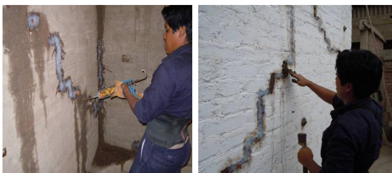
Figure 3. Repair of seismic cracks on a damaged adobe wall. Mud grout was injected in cracks that were opened, cleaned with water, and covered with silicone (left). Wider seismic cracks were filled manually with mud (right).
