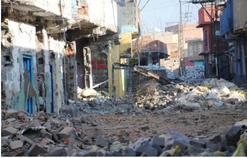
Figure 13. Diyarbakir Sur, after conflicts [32]
