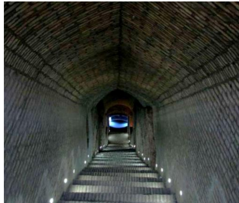
Figure 11. Jame mosque Payab, Yazd [21]
