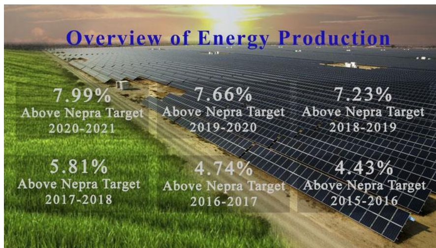
Figure 11: Energy production of QASP Bahawalpur [51]
